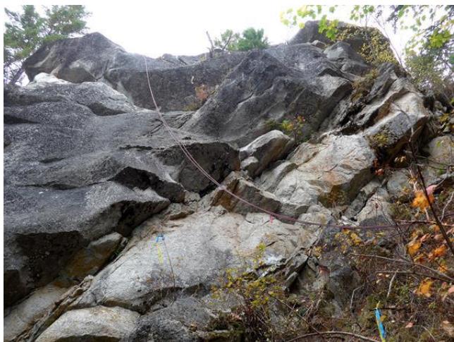
Bear Wall right to Upper Roofs in distance
